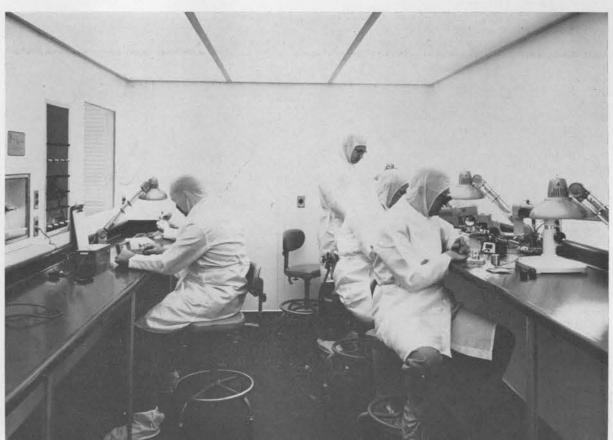
CLEAN ROOM OPERATION and protective clothing worn by technicians is shown in the above photo. The men are performing delicate assembly operations of tiny components requiring dust-free
